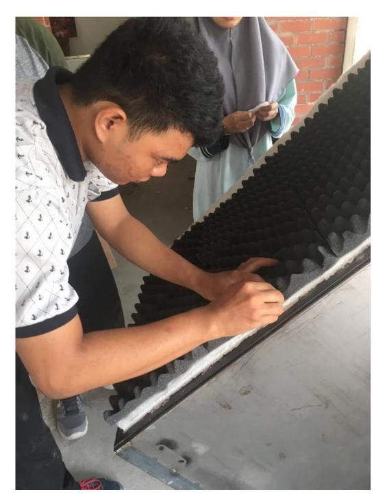
Figure 3.3.4 Mounting the third layer of sound panel, acoustic foam.
