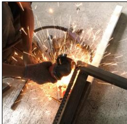
Figure 3.7: Iron cutting proses for plywood structure.
