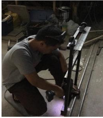
Figure 3.10: Make holes and put bolts and nut
