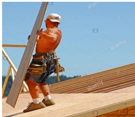
Figure 1.2: show a worker lifting plywood using conventional method
