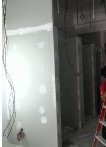
Figure 4.3.3.3 Testing at Shop Lot TTDI Jaya, Seksyen U2, Shah Alam
