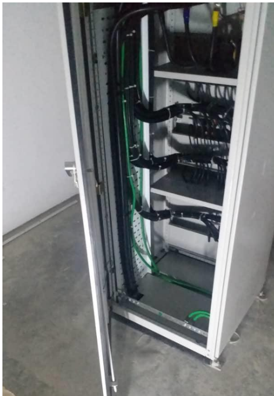
Figure 4.3.4.2 Wiring Work Do by electricians
