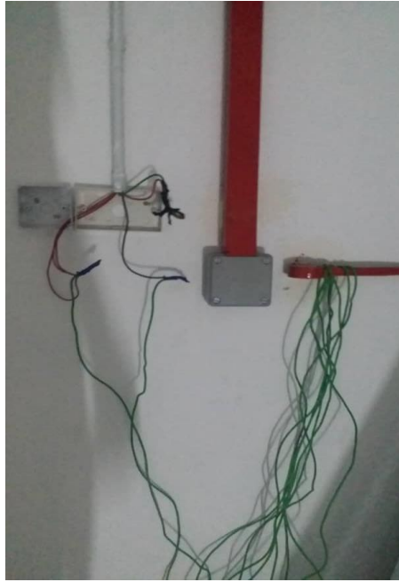
Figure 4.3.3.1 Testing at Shop Lot TTDI Jaya, Seksyen U2, Shah Alam
