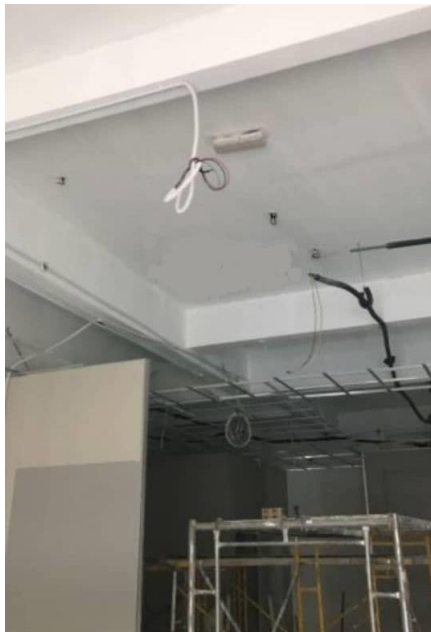
Figure 4.3.3.2 Testing at Shop Lot TTDI Jaya, Seksyen U2, Shah Alam
