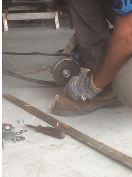
Figure 3.7 Cutting The Steel
