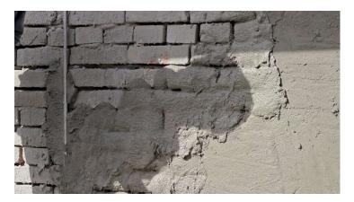
Figure 1: Cement-sand brick wall and plastering
