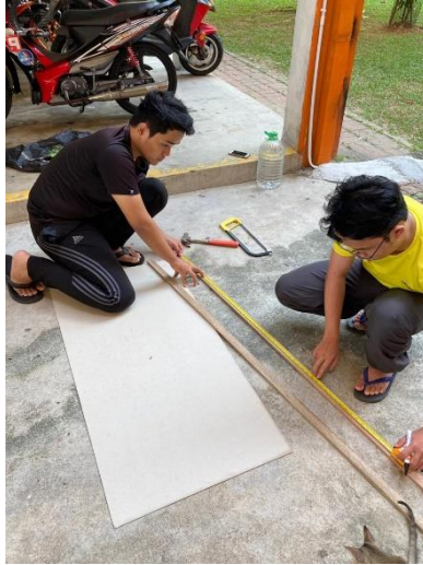
Rajah 1.0 ( Proses membuat formwork/moulding )
