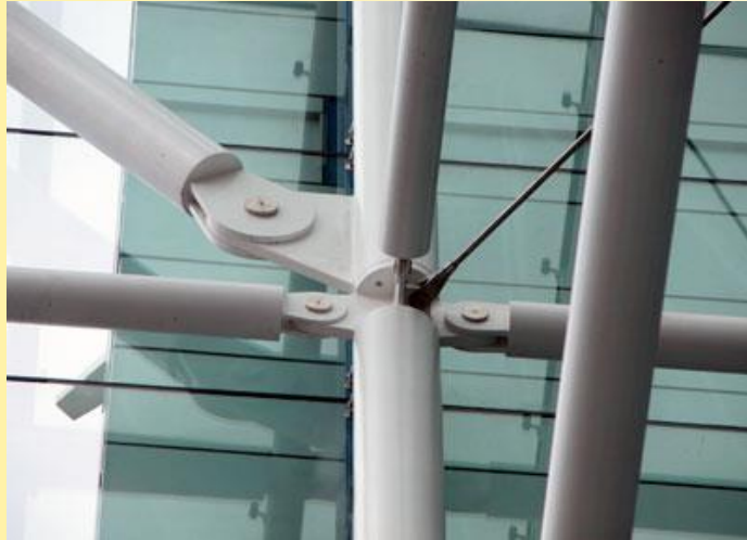
Simple pin connections using two plates
