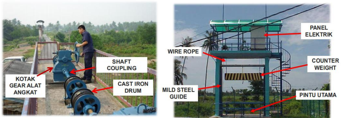
Figure 4.2.3 : Some of water control gate components
