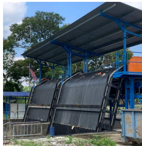
Figure 4.2.2 : Sluice Gate in the rainwater catchment pond
