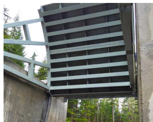
Figure 2.4.5 : Example of Radial Sluice Gate
