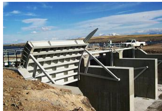
Figure 2.4.4 : Example of Radial Sluice Gate
