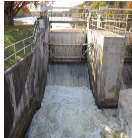
Figure 2.4.3 : Example of Vertical Rising Sluice Gate
