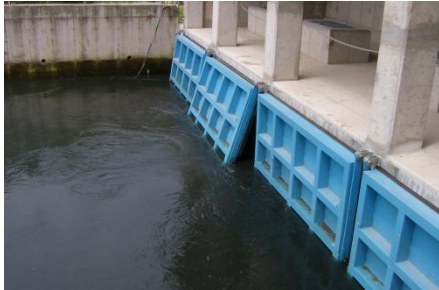
Figure 2.4.1 : Example picture of Flap Gate
