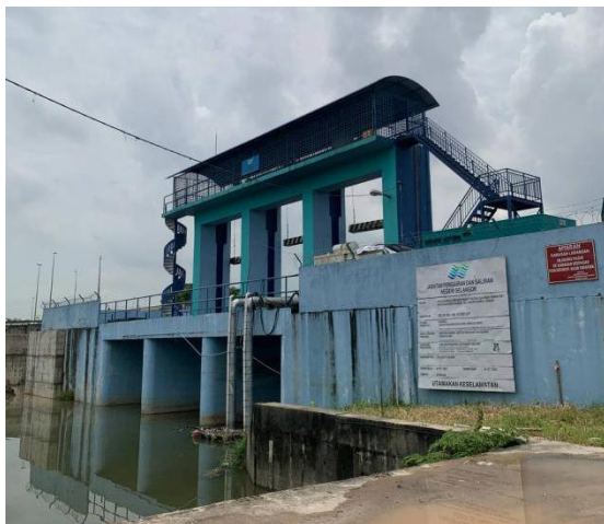
Figure 4.2.1 : The Sluice Gate In Taman Sri Muda
