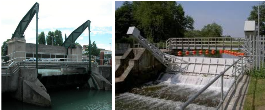
Figure 2.4.6 and Figure 2.4.7 show the example of Rising Sector Sluice Gate
