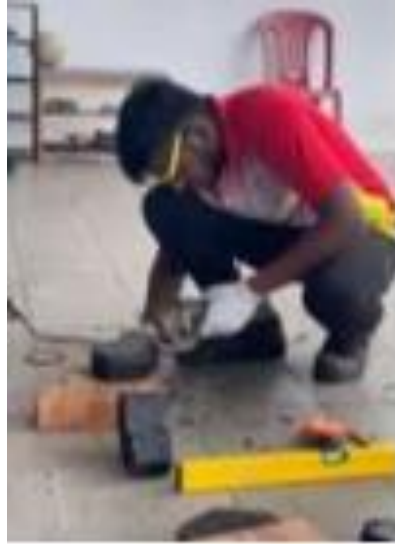
Figure 3.12: Finishing the recycle interlocking brick surface
