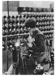
Acetylene welding on cylinder water jacket, US Army 1918
