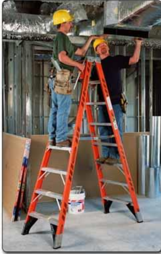
Figure 1.1.2: The Technician Used Ladder to Maintenance the Ducting.
