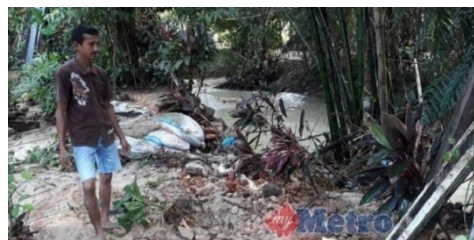
Figure 6: Picture shows that the sandbag are broken
