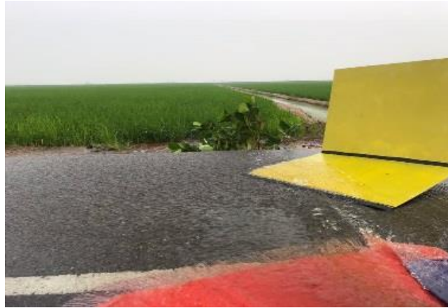
Figure 2: The flood barrier was used to change the flow of water beside paddy field
