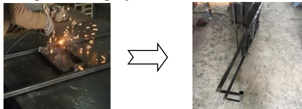
Figure 3.4.12: welding for front part
