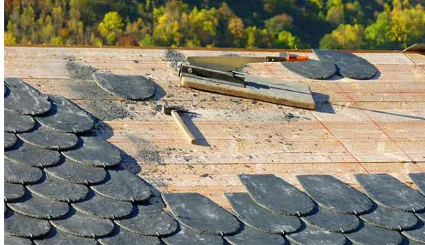
Figure 2.0: wood shingles being replaced by wooden shingles
