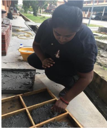
The concrete mixture is compacted.
