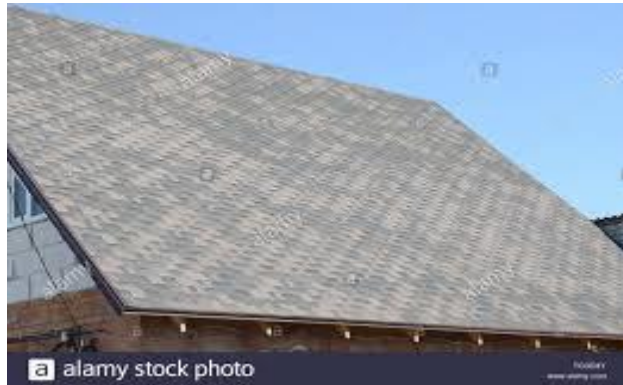
Figure 2.1: example of bituminous tiles that has been fixed in a roof of the house
