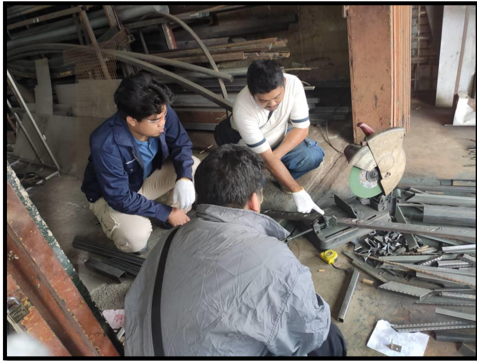
Figure 3.6 The start of the assembling process
