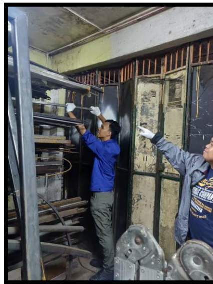
Figure 3.3 Handling the circular hollow tube
