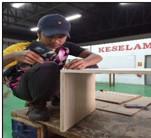
Cabinet installation process
