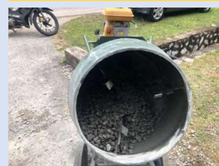
2. Put all materials in concrete mixer.
