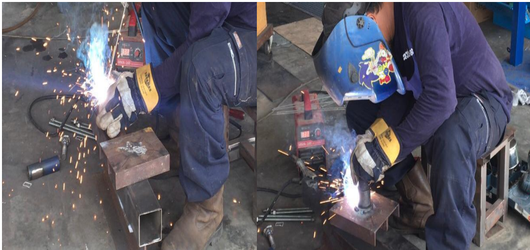
Rajah 3.13: Kerja kimpalan
