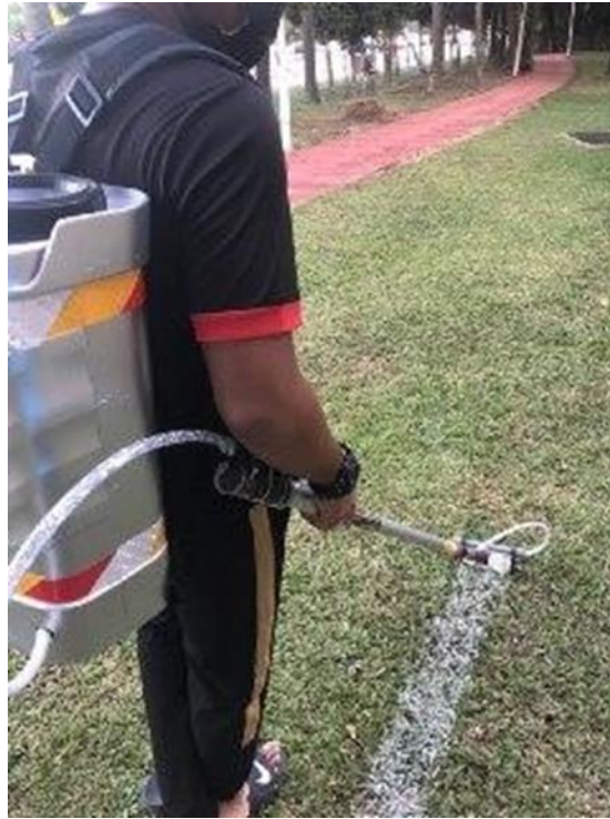
Figure 4.4.5 Line Marking Work
