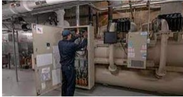
Figure 1: Technician perform minor repairs for chiller
