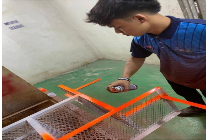
Image 3.5 (n) Showing painting the structure.
