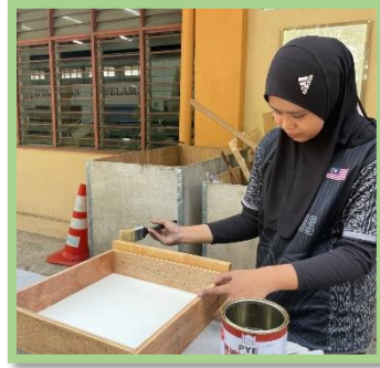
Figure 3.10: Applied shellac to all cabinet surfaces and drawers.
