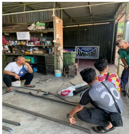
Figure 3.7 Cutting The Steel
